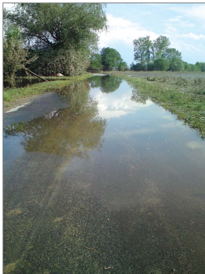
Zalana droga Flooded road
